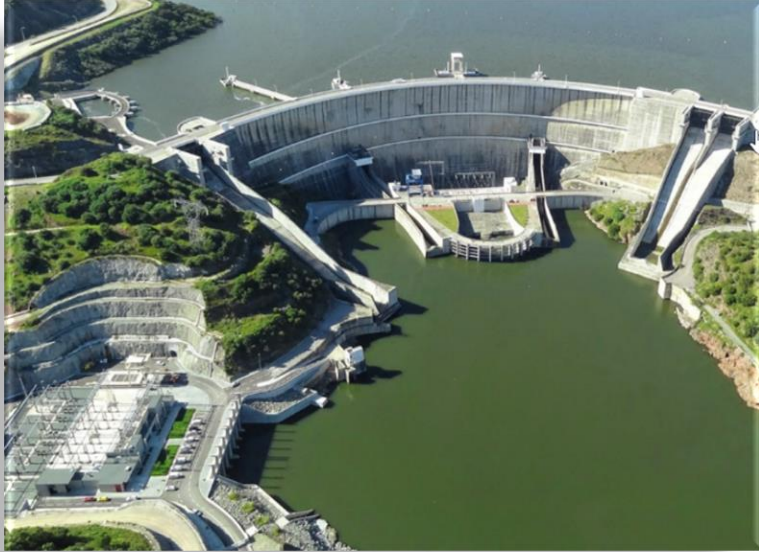
ALQUEVA II HPP 2 x 125 MW Pump-Turbine
