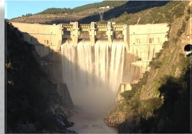
FOZ TUA HPP 2 x 135 MW Pump-Turbine
